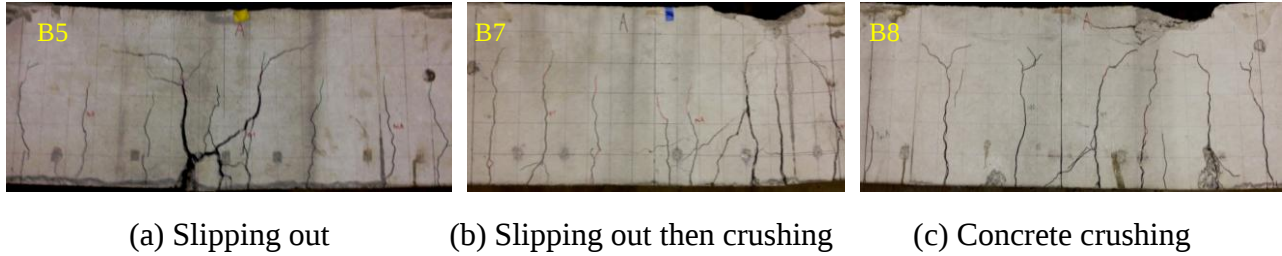
Figure 7: Failure modes of beams
