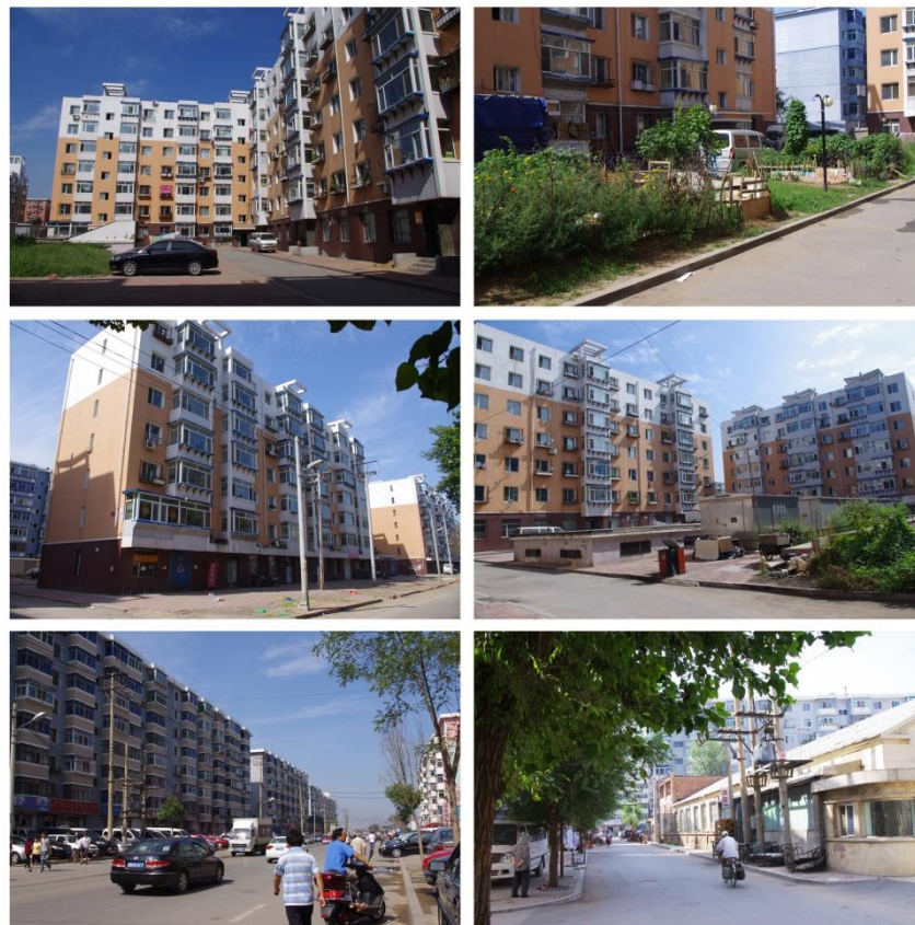
Figure 3-3 Environment in the Xianggongbei project and the surroundings
