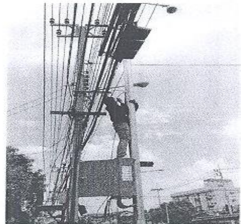
Picture 5.1 the Installed Housing of Telecommunication Networks and CCTV at the Intersections
