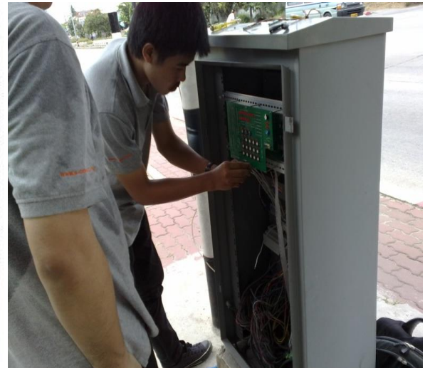
Picture 5.1 the Installed Housing of Telecommunication Networks and CCTV at the Intersections
