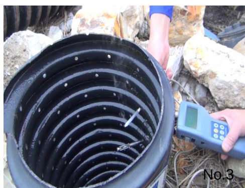
(a) Outflow vent (No.3)
