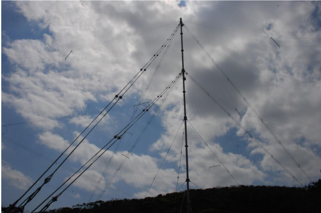
Figure 1.9. Delta-loop antenna of ionosonde station at Ohgimi, Okinawa.
