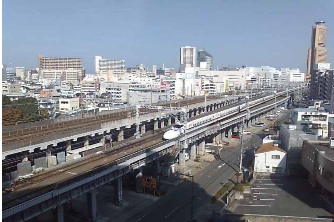
Fig. 1.4 High-speed train running on the viaducts [8]
