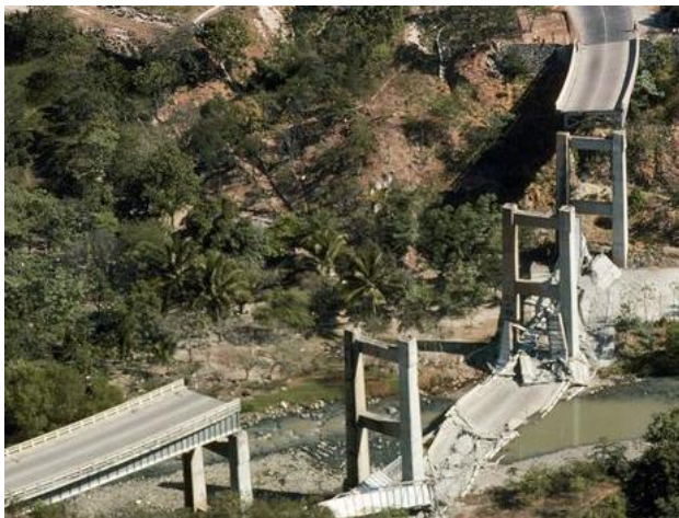
Fig. 1.3 The falling down of deck in earthquake
