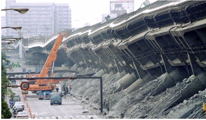
Fig. 1.1 The collapse of a bridge in Kobe earthquake
