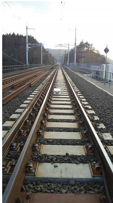
Figure 16 Narrow gauge and standard gauge tracks
