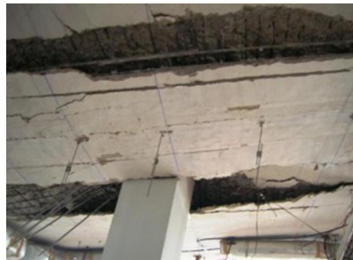
Fig. 1.2 Combined FTC damage and fatigue loading
