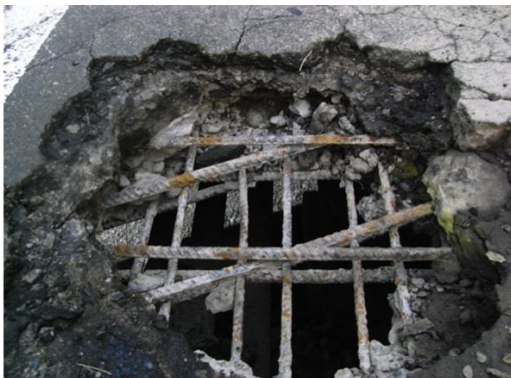
Fig. 1.2 Combined FTC damage and fatigue loading
