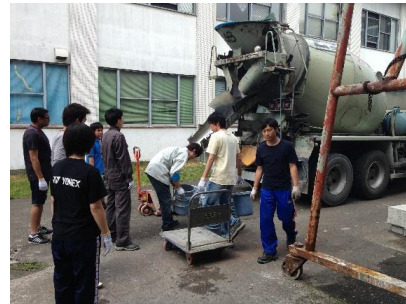
Casting of concrete
