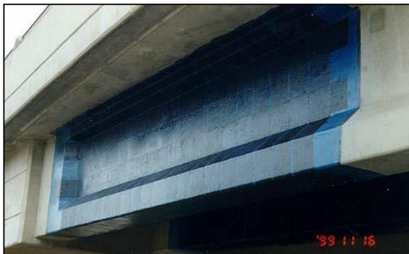
Figure 2-6 Shear strengthening of bridge girder
