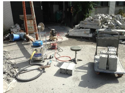
Surface preparation by disk grinding
