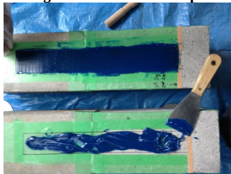
Put first coat of the resin
