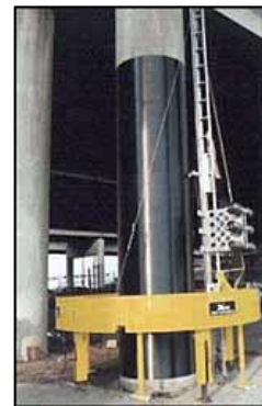
Figure 2-7 Axial strengthening of bridge piers
