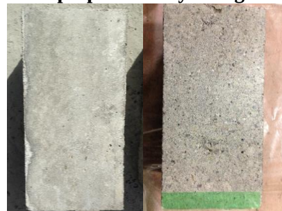
Concrete surface before and after preparation
