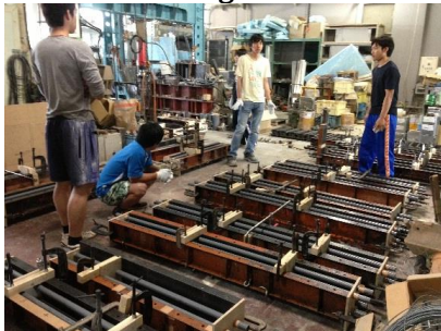
Preparation of formwork
