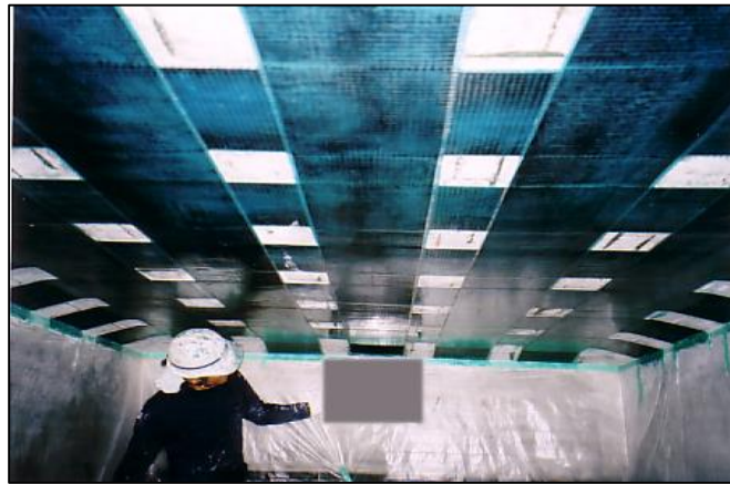
Figure 2-5 Application of CFRP for flexural strengthening of bridge decks
