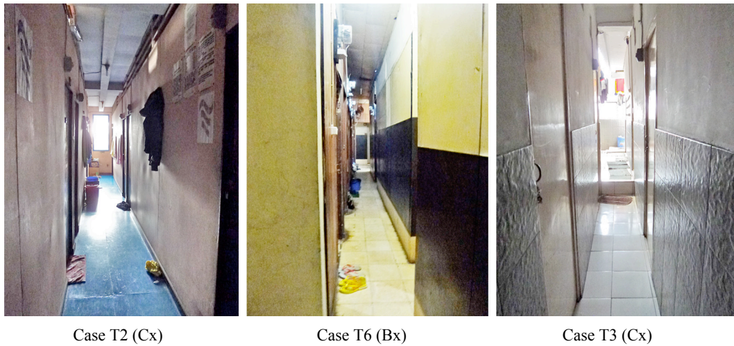
Fig. 6.4 Example of long and narrow double-loaded corridors found in surveyed kots
