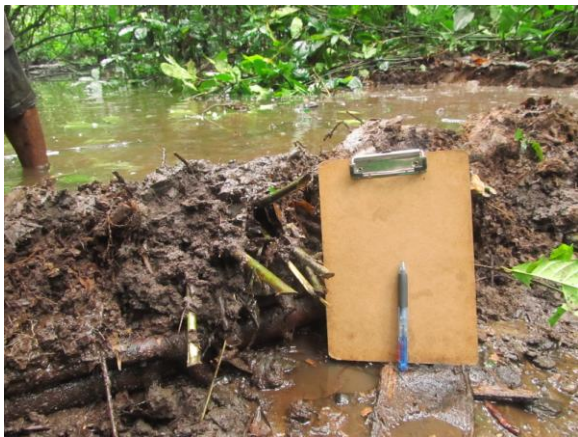
Figure 17 : A 20-30 cm height of soil wall that was constructed to hold back a shallow river temporarily.
