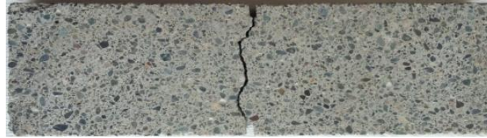
(a) For non-damaged specimen and specimen without fire crack
