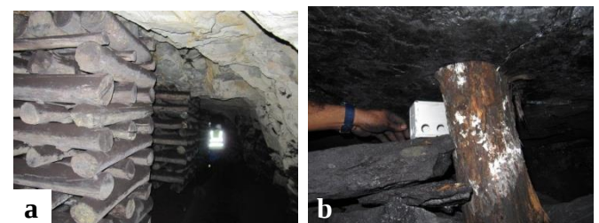
Fig. 3. (a) Lower seam adit in Mchenga Coal Mine (b) Data logger fixed in position close to the coal bearing rocks.
