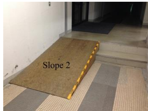
(b) Upslope and Stairs
