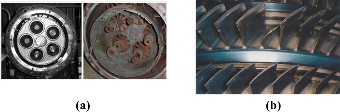
Fig. 1.19 Damage of industrial burner system; (a) burner nozzle assembly and (b) Turbine blade/Bucket.
