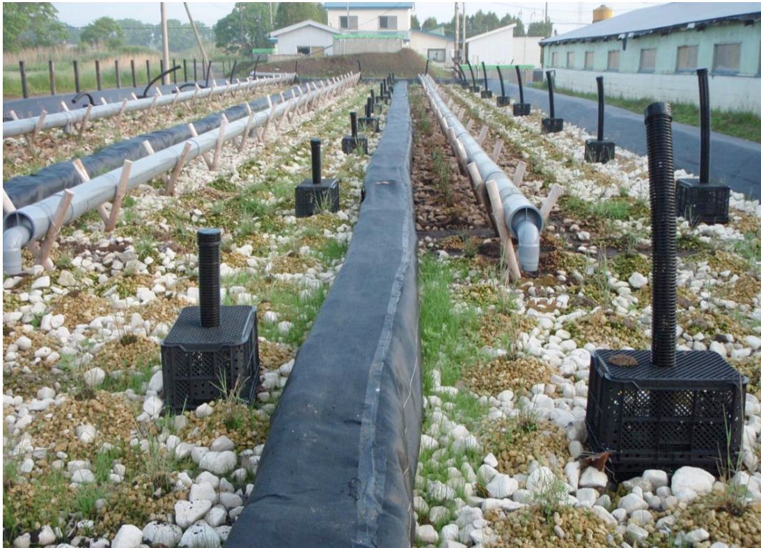
Fig. 2-3 Surface partition and reinforced safety bypass.
