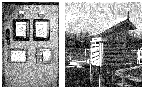
Fig. 4. Analog recorder (left) and instrument shelter (right) in 1966. Daily maximum and minimum values were read from the chart.
