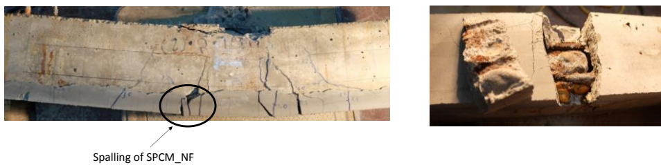
Figure 3.17. Spalling of non-fiber containing SPCM
