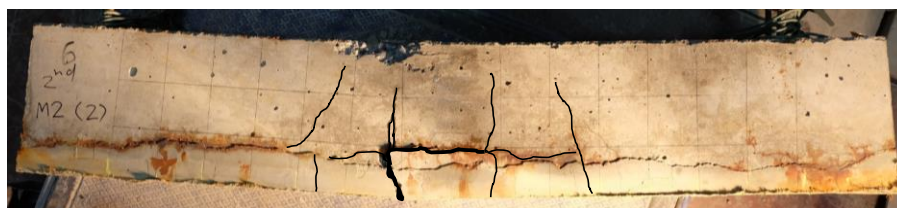
(a) The beam repaired with method 2
