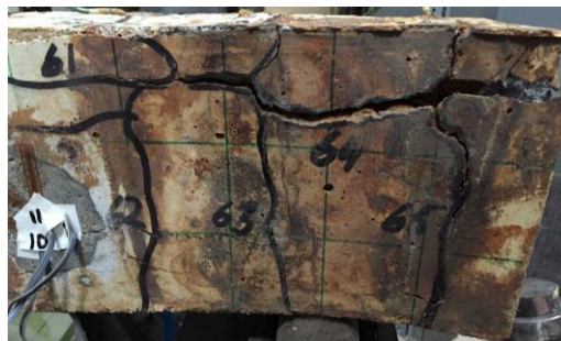
Figure 3.41 Formation of cracks during bending test of B17S-FS-13/80
