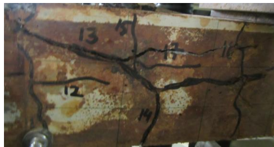
Figure 3.43 Formation of cracks during bending test of B23S-MS-13/120
