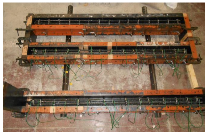
Figure 2.7 Formwork and other preparations for casting of concrete beams
