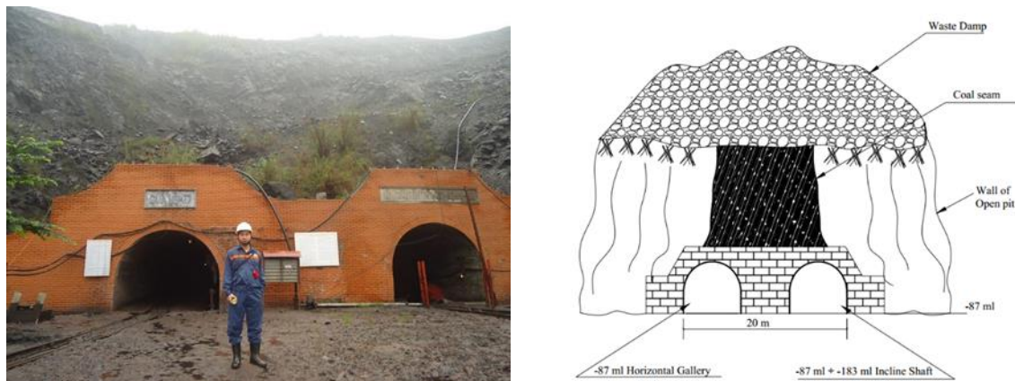
Figure A2-6: Pit mouths Khanh Hoa Coal Mine driven from the outcrop wall of coal seam No. 16 after finishing the open pit mining.
