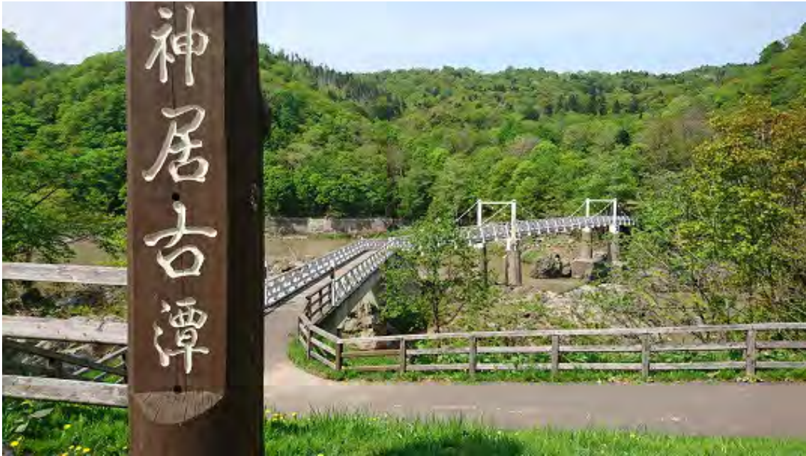
Figure 7: Kamuikotan Suspension bridge (accessed 06/09/2018: http://map.uu-hokkaido.jp/e/asahikawa-kamuikotan/ , CEDARS Communications Co. Ltd.).
