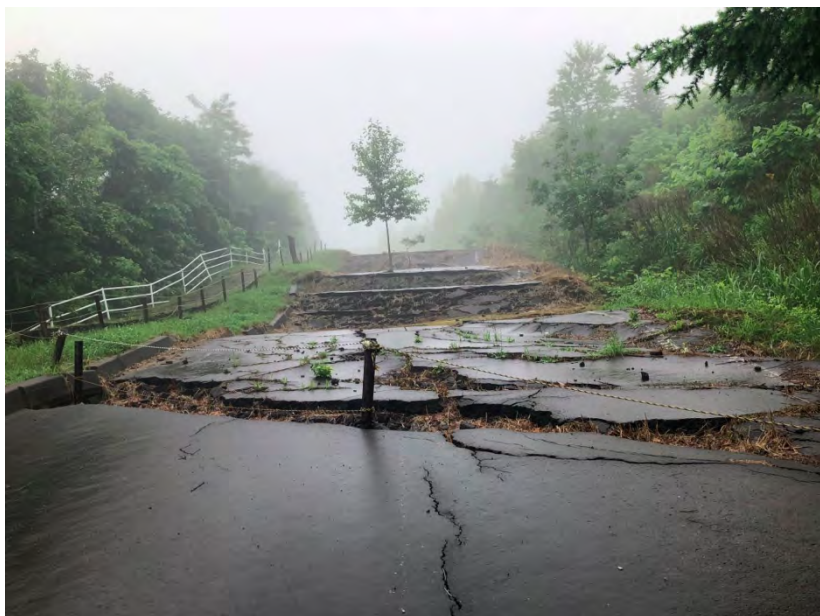
Figure 30: Nishiyama Crater Walking Trail - Road disrupted during the Mt. Usu’s latest 2000 eruption.
