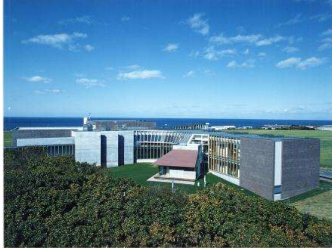
Figure 3.3. The NIHORU exchange center in Nemuro
