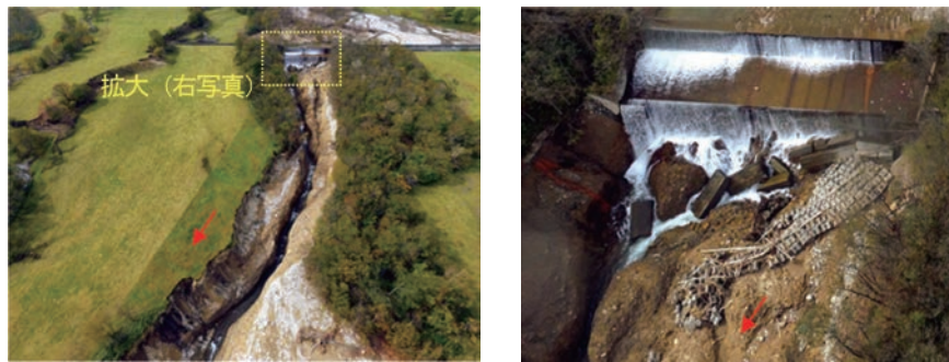
写真-12 3号砂防堰堤損傷状況 (UAV による斜め写真) Photo 12 The damage of No. 3 check dam (Photo taken by UAV)
