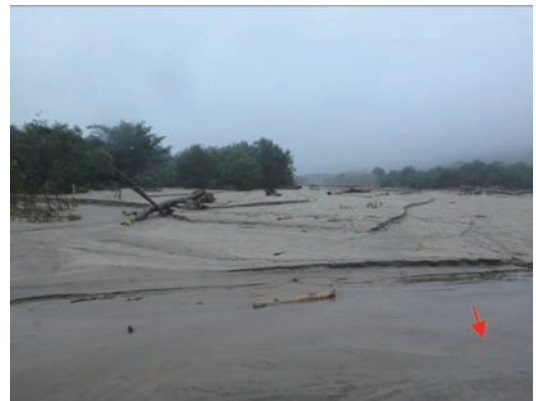
写真-6 2号砂防ダムの土砂・流木の堆積状況 Photo 6 Sediment and drift woods at No.2 sabo dam
