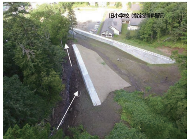
写真-12 導流堤による導流状況 Photo 12 The training dyke at the Shogakkonosawa
