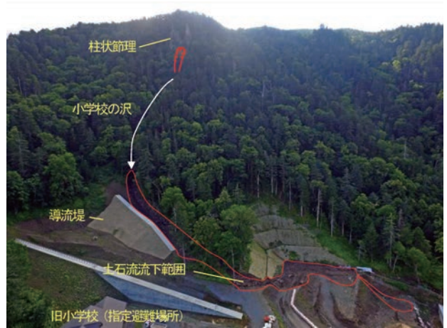
写真-11 小学校の沢全景 Photo 11 Aerial view of Shogakkonosawa catchment
