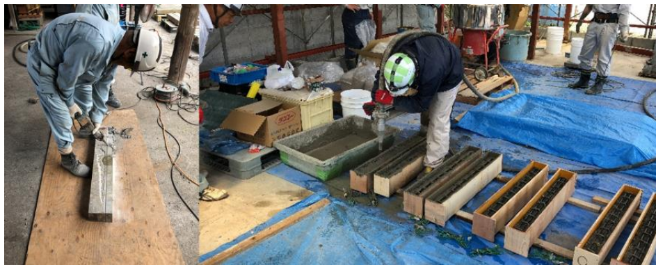
Figure 2.8 Removal of concrete cover and spraying PCM on RC beam.
