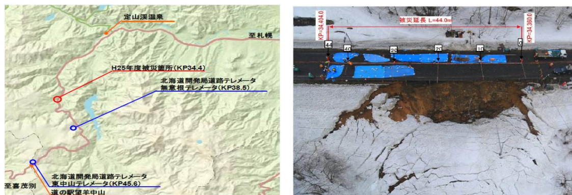
Figure 2.6 (a) Location of slope failure (b) slope failure covered with snow.
