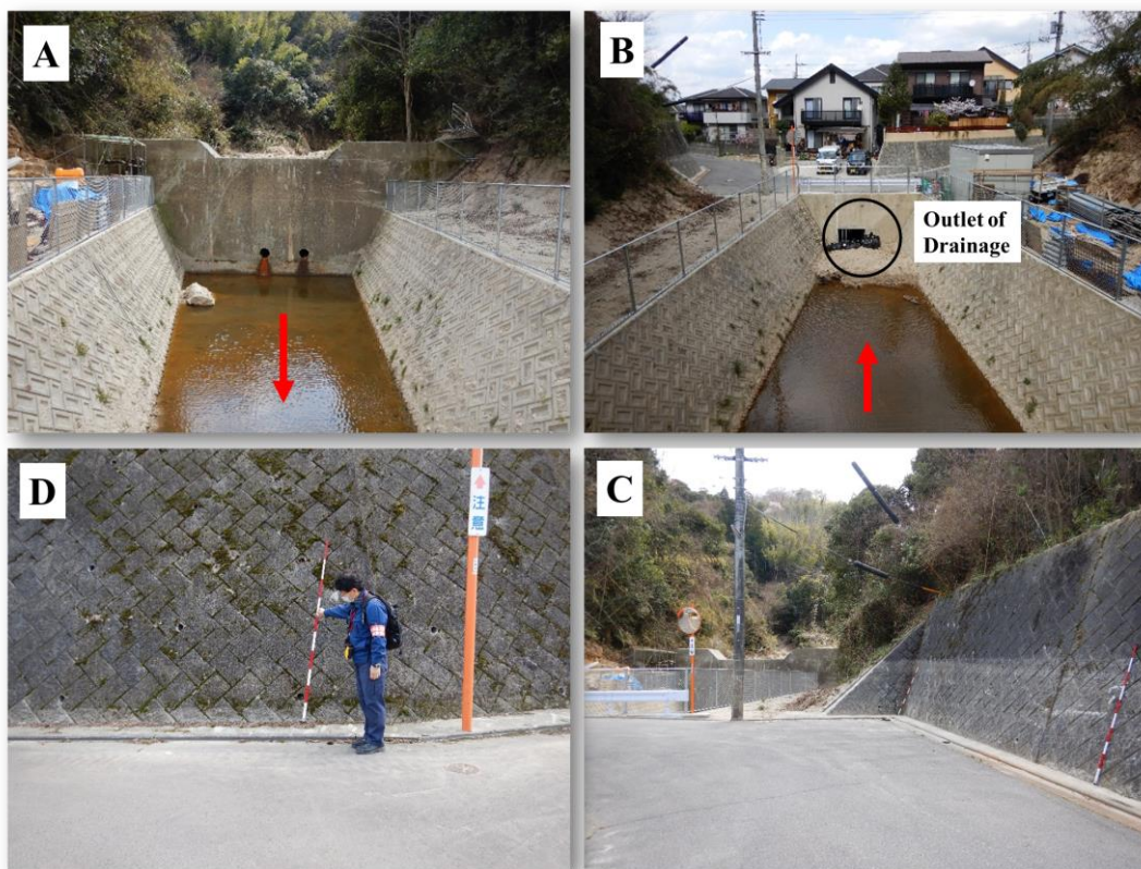
Fig. 3-5. Sediment retarding area and actual situation of damaged from SSF
