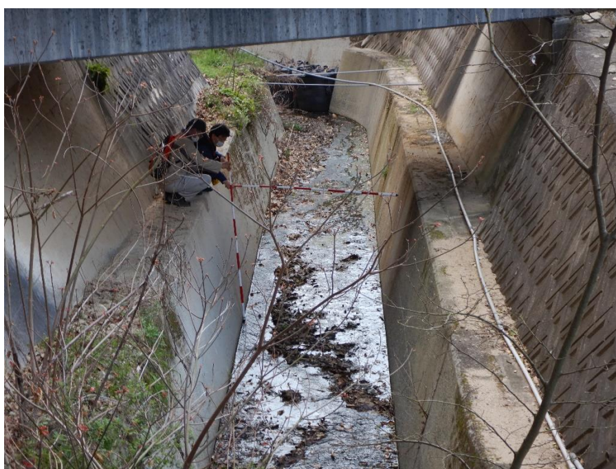
Fig. 3-11. Measuring a scale of drainage
