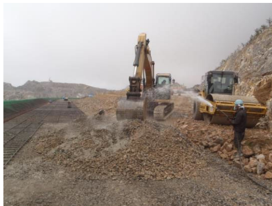
(c) The area of cement reinforcing on the front side of rock piling.
