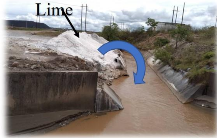
Fig. 6.2. Un-mechanised wastewater treatment without pH monitoring and control
