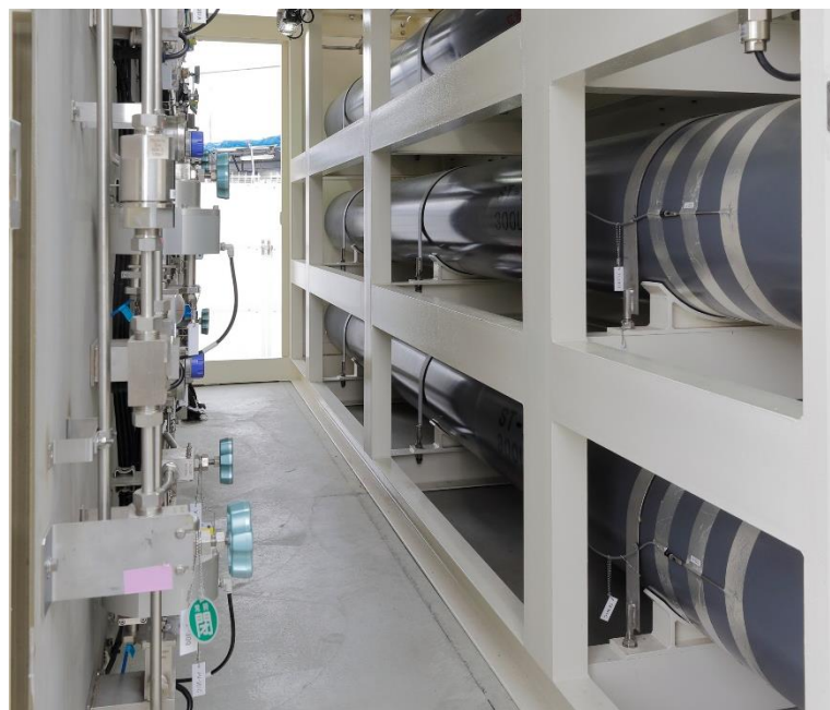
Fig. 1-5 Hydrogen storage tanks at refueling hydrogen station.
