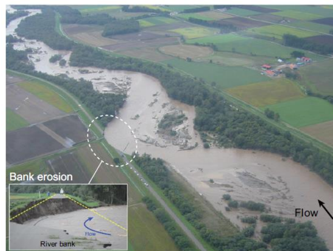
Figure 1.2. Bank erosion disaster happened in Otofuke river, 2011 (Otofuke River, Japan, Nagata, 2014)
