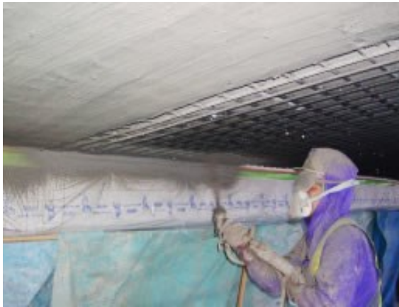
(a) Spraying [Nara Construction Co., Ltd.]
