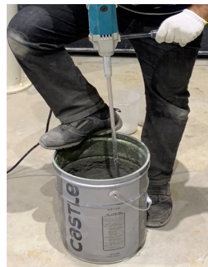
(c) PCM mixing by hand mixer
