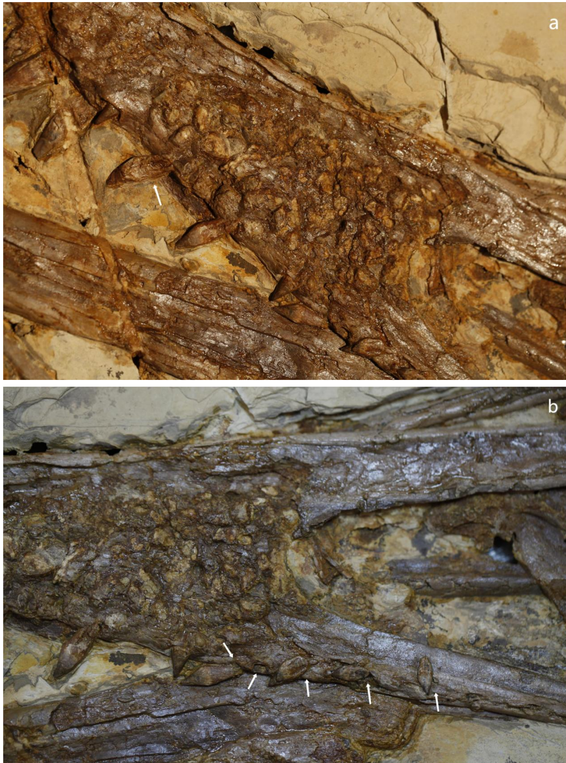
Figure 49. Details of pathological damaged area .
