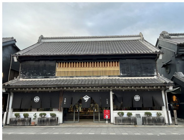
Figure 3: The Ōsawa residence, Kawagoe. Photo: Toyozawa Chikako
