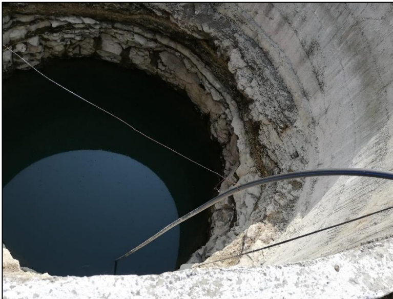
(b) Underground water extraction from the well
