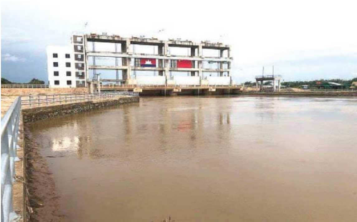
Figure 3-4 Kang Hot headwork site
