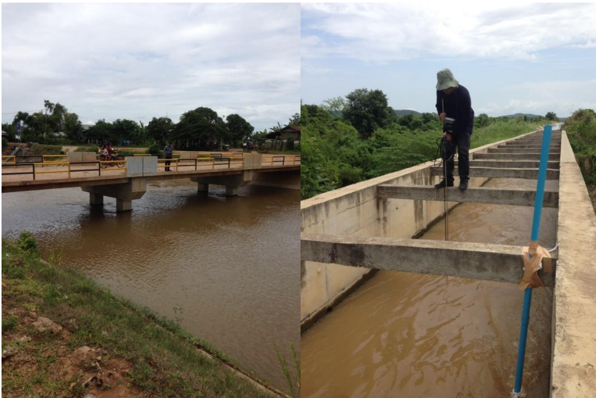
Figure 4-5 Canal discharge measurement using the Current Meter at the Right and Left main canal.
