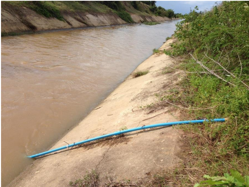
Figure 4-9 Installation of water level logger at the left main canal
