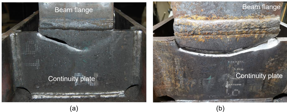
Figure 3.21 Fracture in the continuity plates of Specimens: a) W1, and b) W2.
