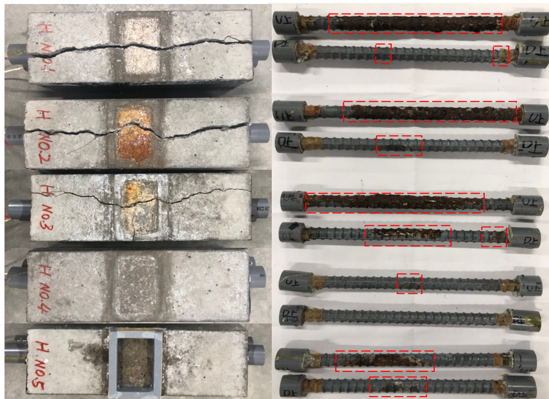
(a) Appearances of H concrete ( H1, H2, and H4 on 1051 days; H3 on 692 days; H5 on 799 days), rebars on the split date
