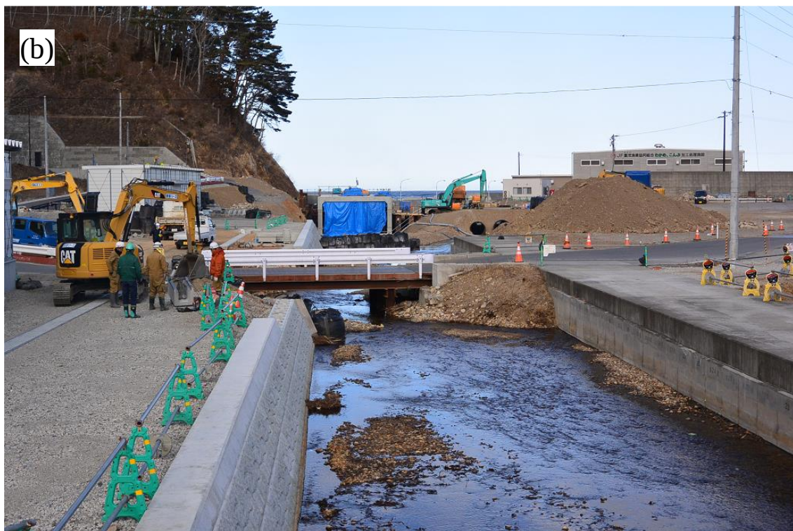
Fig. 5-1. View of the lowest reach of the Otohe River. Before (a: May 19, 2014) and after (b: March 7, 2022) river alteration.
