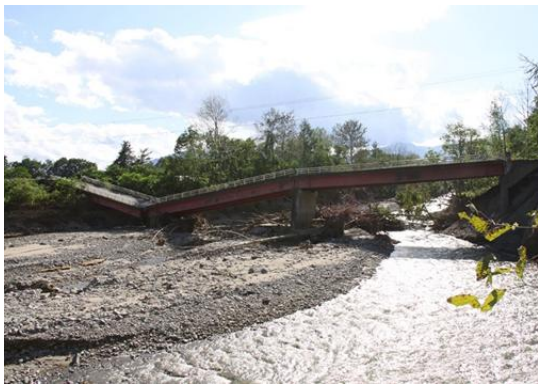
(a) Kamimemuro Bridge
