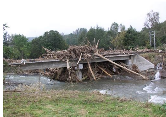
(b) Simoshintoku River JR Bridge
