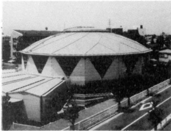
Figure 2.2 Vibration test on a full size suspen-dome (source: Tatemichi et al. 1997)
