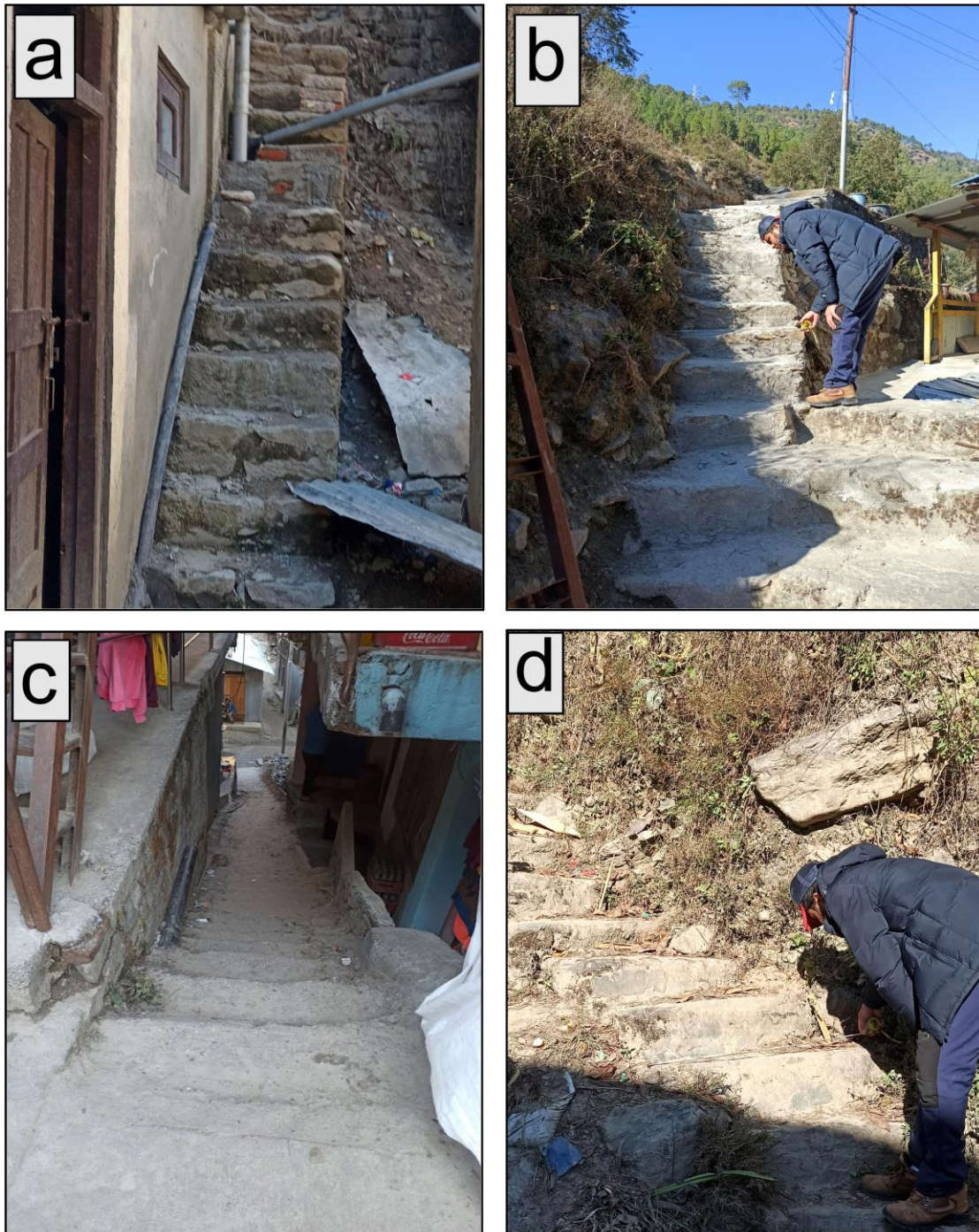
Figure 4.9 Existing evacuation routes in Singati. a, b, c and d are close-up photos of the existing evacuation route. See Figures 4.8 for locations (photos: Bikram Parajuli)
