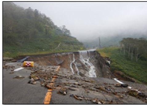
(a) Geotechnical disasters in Hokkaido, Japan induced by heavy rainfall on August, 2016
