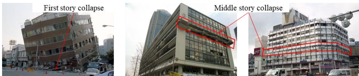
Figure 1.1 Examples of building story failure during earthquake
