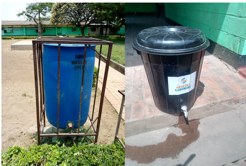
Figure 3 | A water tank and handwashing point.
